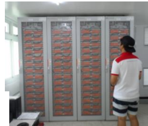
LITHIUM BATTERY, 273KWH
