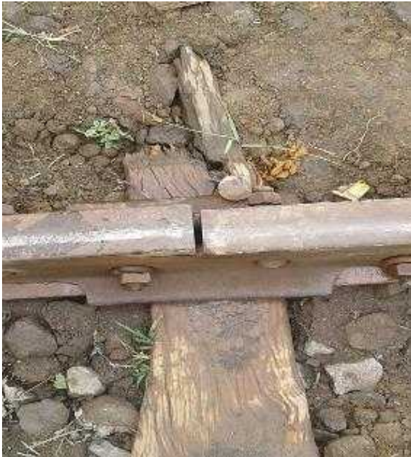
Damaged rail track in Laguna
